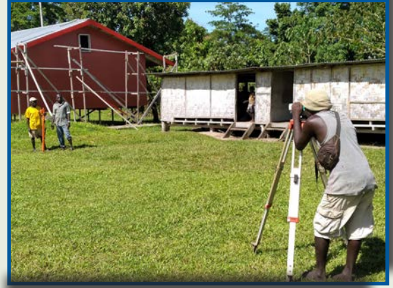
Above: Local community hard at work
