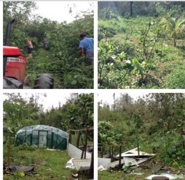
Extensive damages to the Tutu Rural Training Centre
